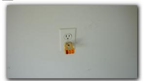
1 All electrical receptacles installed in garages are required to be GFCI protected.
