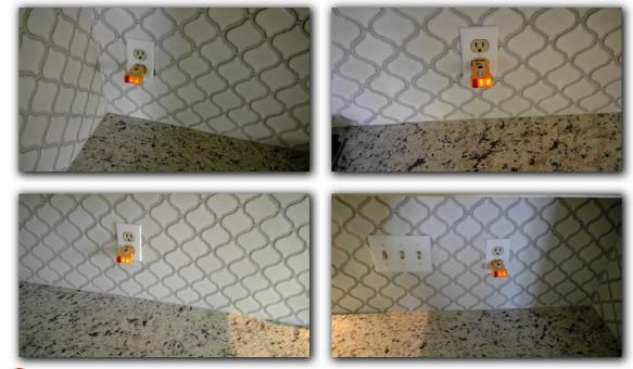
1 All receptacles in the kitchen area are required to be GFCI protected with the exception of receptacle designated for refrigerator.
