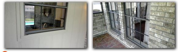
**1** The TREC Standards of Practice instructs inspectors to report as deficient: Missing or damaged window screens.
