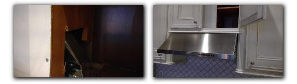
1 The exhaust duct is not connected to fan and cooking exhaust is blowing into cabinet above vent hood.
