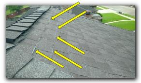
1 The edges of shingles are showing wear with exposed fibers.
