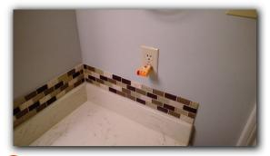
1 All electrical receptacles installed in bathrooms are required to be GFCI protected.
