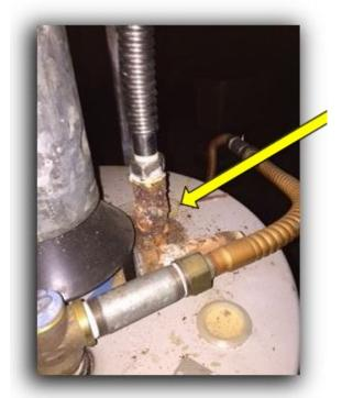
1 This nipple is in very bad condition and could start leaking water any time. Need to replact this nipple ASAP to prevent water damage. The corrosion is due to galvanic corrosion from dissimilar metals. A dieletric nipple should be installed to prevent further corrosion.
