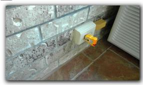
1) All exterior electrical receptacles are required to be GFCI protected.
