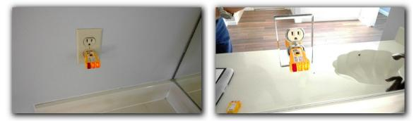
A The hall bathroom electrical receptacles are not GFCI protected.
