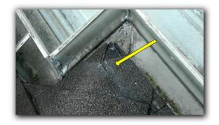
▲ Damaged shingles on the Front side of house.
