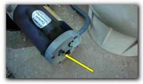
Mater leaks noted at swimming pool filter and pump equipment.
