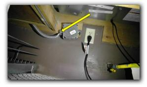
The exterior electrical receptacles are not GFCI protected receptacles.
