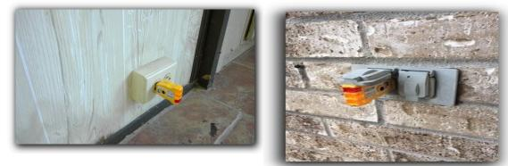
A The electrical receptacle on Left wall of patio is not working.
