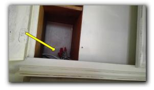
Conduit not secured to junction box, in cabinet under gas cooktop. Receptacle in cabinet under cooktop not GFCI protected
