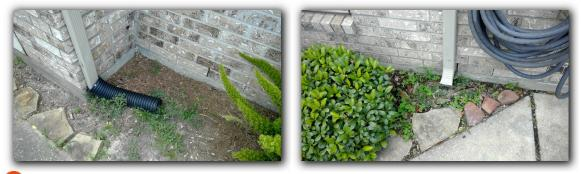
**1** Rain water discharging from roof gutter system should be discharged, where possible, 5' away from foundation.
