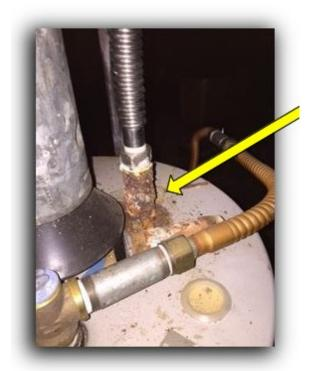
1 This nipple needs to be replaced ASAP before water damage occurs.
