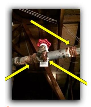
1 This piping should be replaced ASAP to prevent water damage.
